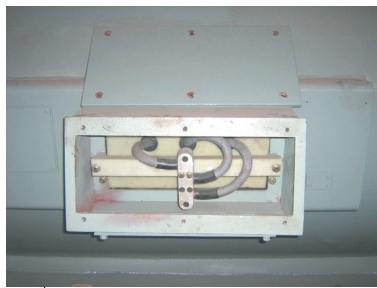
Fig 9 : Typical Alternative Arrangement for Neutral Point Termination
